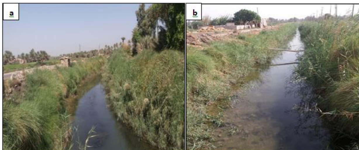
Fig. 3 : a. Aljbsa drainage; b. Aljharh Algerbeah drainage.
